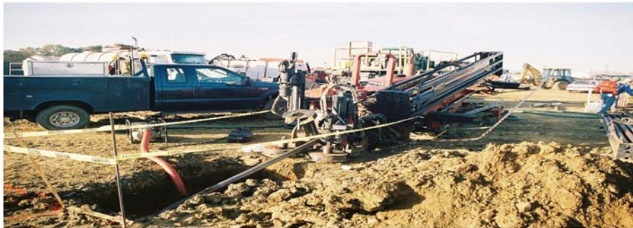
FIGURE 3. Directional drill rig.
