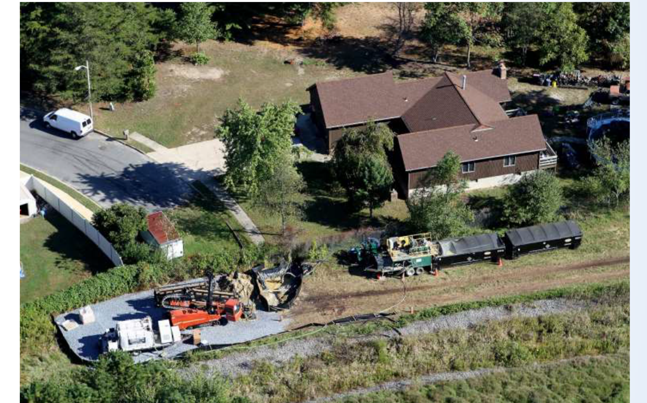
Drone Fly Over of Staging Area and Drill Entry
